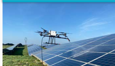
SOLAR PANEL CLEANING
